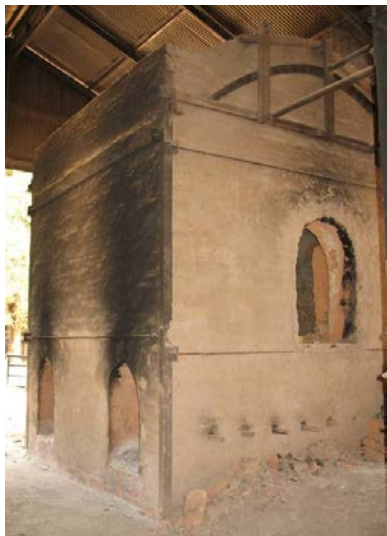
Figure 4.5 Kiln showing doors to fire chamber bottom left, filter element chamber right
