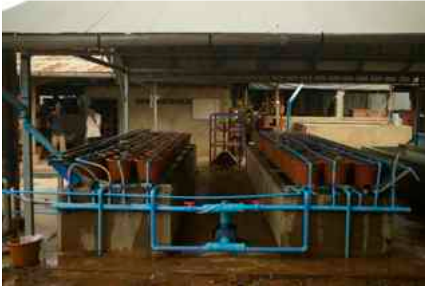
Figure 4.20 Recirculating continuous flush system for arsenic leeching
